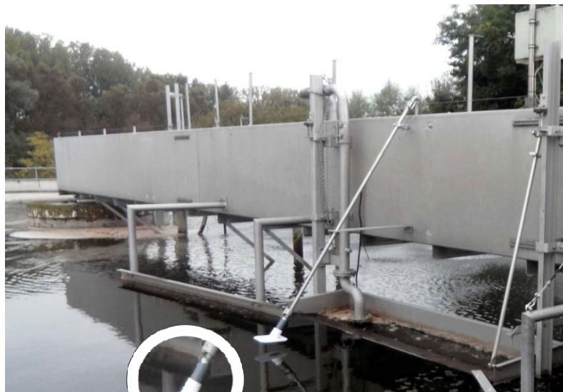
Surface scanner for secure detection of float sludge.
