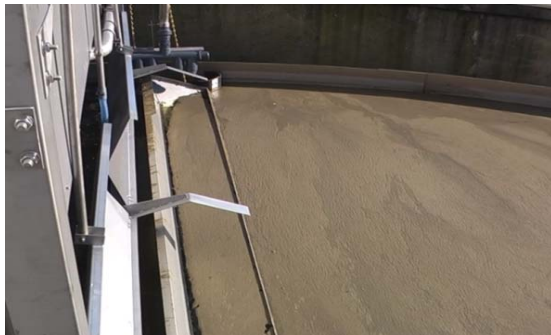
3. Now follows a controlled hydraulic separation from the water surface
