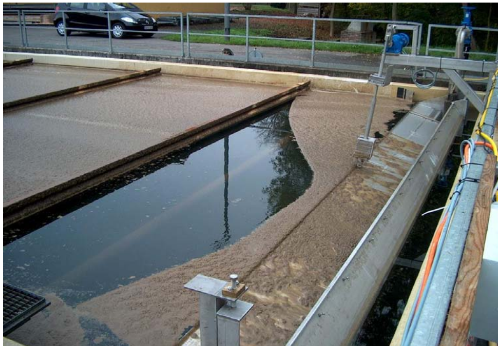
"Suction effect" of a fully automatic, self adjusted skim channel
